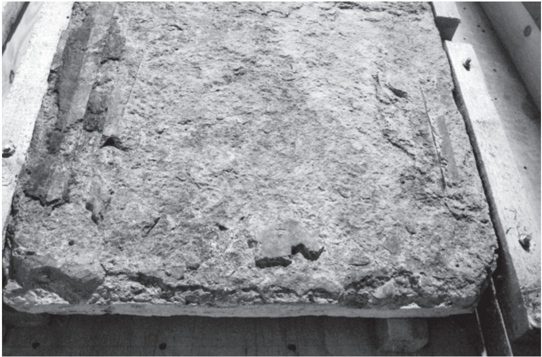
Fig. 9. Detail of the indent in the shrine base of St. Thomas Cantilupe, Hereford Cathedral, showing trimming to the slab. (photo © Sally Badham)
